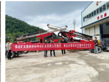
紫金矿业河南某金矿 断面2.6m×2.4m/2.6m×2.6m
